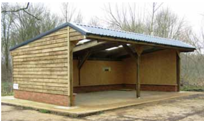
The new Jack Crawley Memorial Barn, home to the Flit Valley Heritage Discovery Centre.
