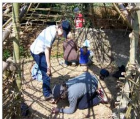
The roof starting to come together
